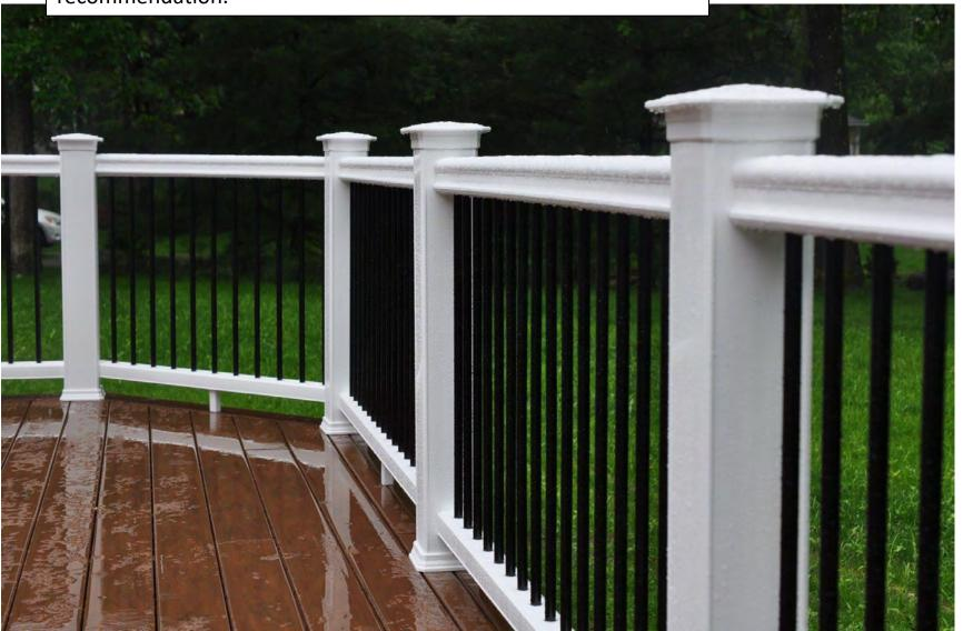
Below is an all-aluminum handrail, upper and lower handrails and balusters are all aluminum. Aluminum tends to scratch, bend and dent more easily than composite. My least favorite choice for commercial applications.
